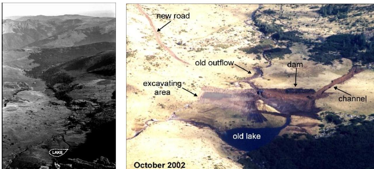
**Fig. 1.4.1.** Left: Lake Stiol on 21<sup>st</sup> September 1975 (photo: Pascu D.). Right: Construction works at Lake Stiol on the 3<sup>rd</sup> of October 2002 (photo: Goja L.).
